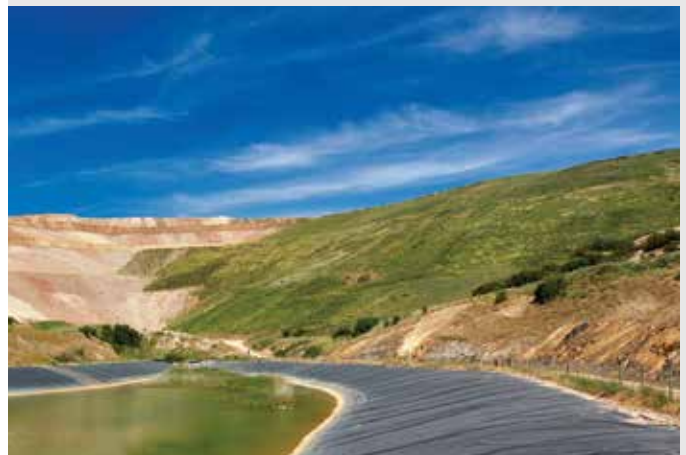
Water collection and reclamation in progress at Kışladağ, Turkey
