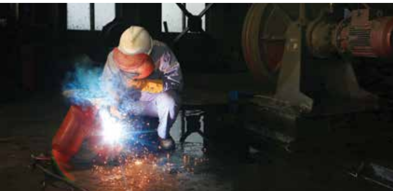
Welding at Tanjianshan, China
