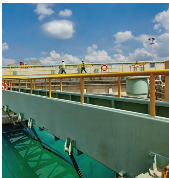
Kışladağ water treatment plant.
