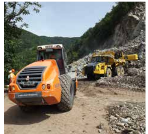
▲ Site preparation work at Certej, Romania.
