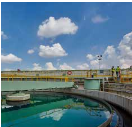
Water treatment plant at Kışladağ, Turkey.
