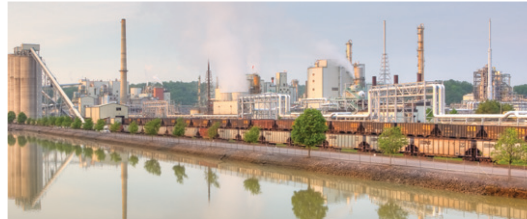
Eastman Chemical Company's coal gasification facility is located in Kingsport, Tennessee.
