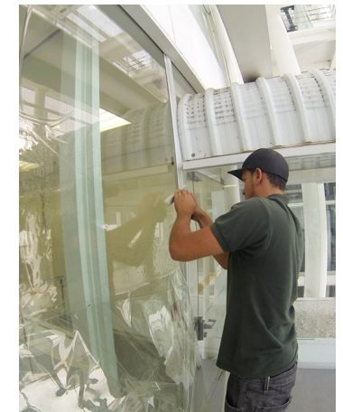
Installation of LLumar® window films at Petrobras in Brazil.
