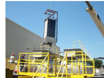
Installation of the new membrane bioreactor at Eastman's Maua, Brazil, site.
