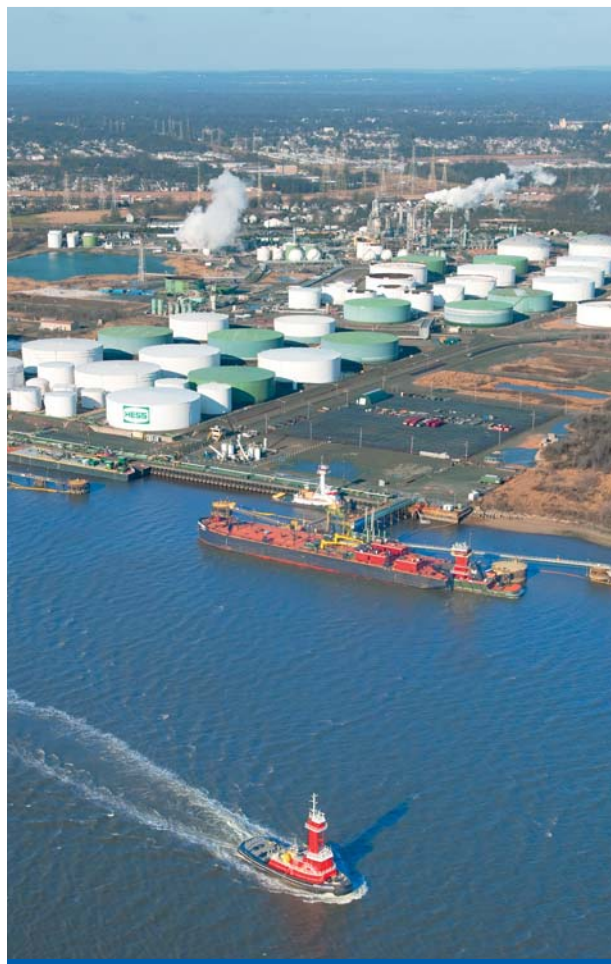
Port Reading Refinery, New Jersey
