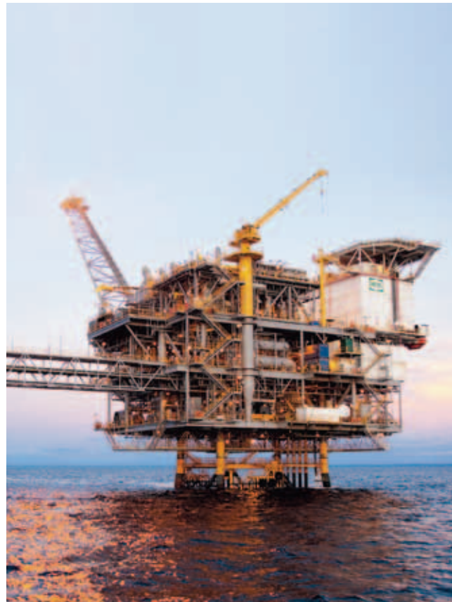
Okume Production Platform, Equatorial Guinea
