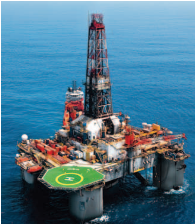
Drilling Platform, Australia
