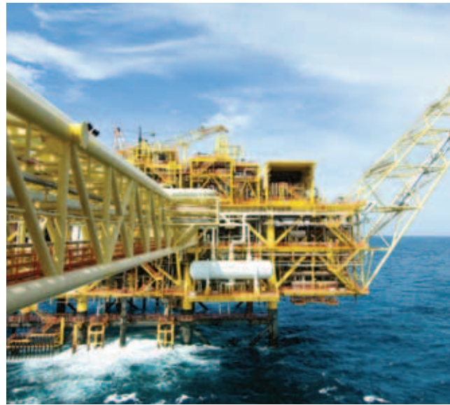
Production Platform, Malaysia/Thailand Joint Development Area
