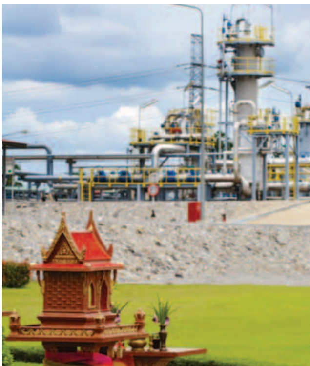
Gas Plant, Sinphuhorm, Thailand
