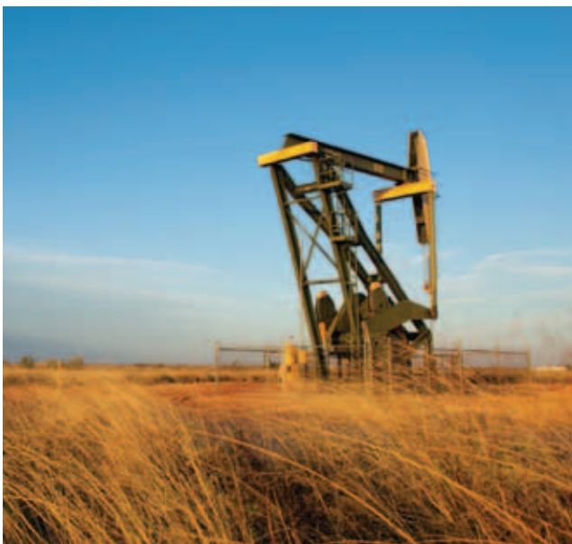
Production Rig, Seminole, Texas
