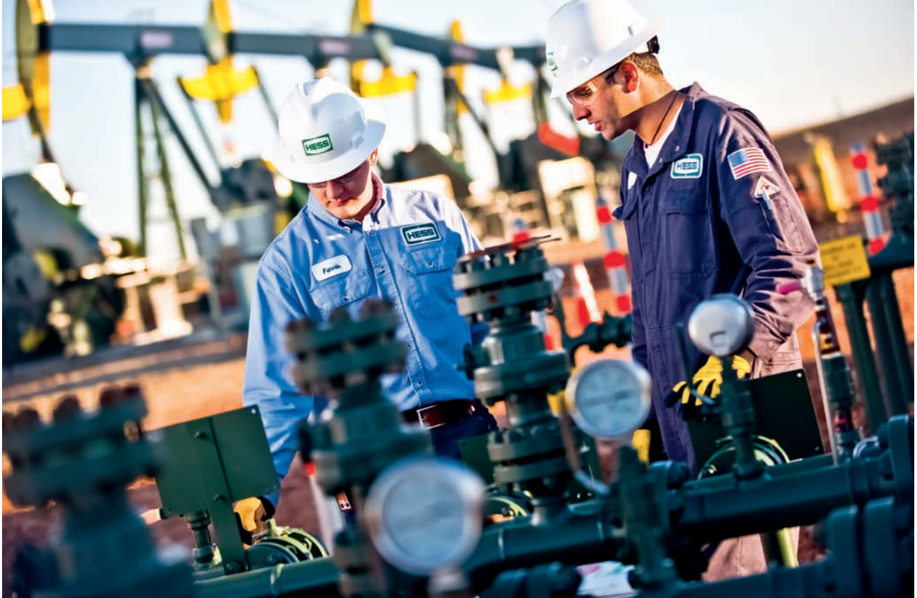
Drilling Operations, North Dakota
